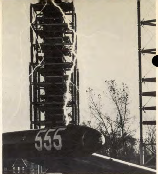
FIG. 13 Simulated lightning tests on wing-tip fuel tank at the GE High Voltage Laboratory, Pittsfield, Massachusetts.
