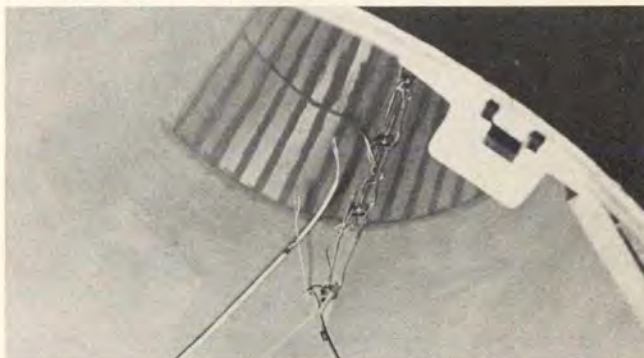
Typical lightning damage to pitot static lines and heater power cord
